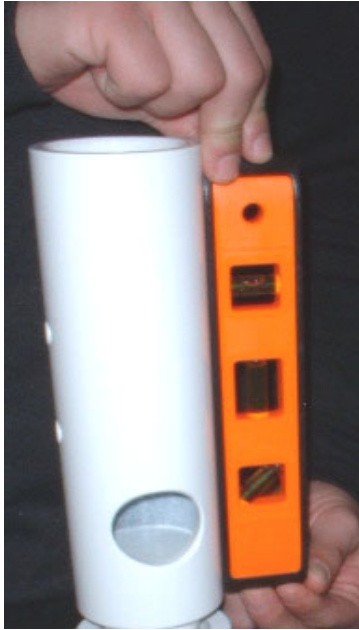
Leveling the unit mounting post.
